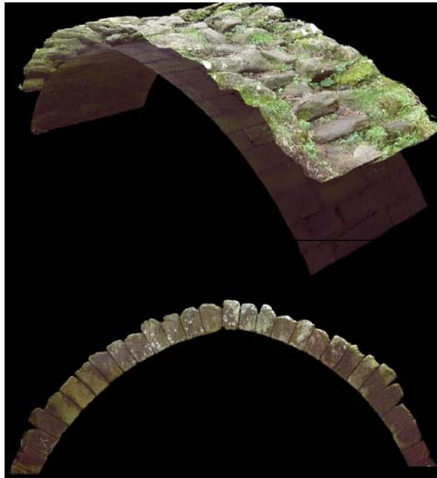
Fig. 2. (a) 3D point cloud model of the Xuño Bridge showing the irregularity of stone's thickness through the whole width of the arch (b) Upstream view of one slice upon the arch of Xuño Bridge showing diversity of the stones shapes and position of the real contact interfaces
