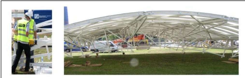
Figure 1. Arched prestressed trusses in Hyde Park, London
